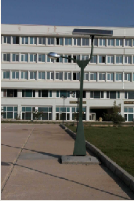
MUGLA UNIVERSITY STREET LIGHT-PV PANELS
