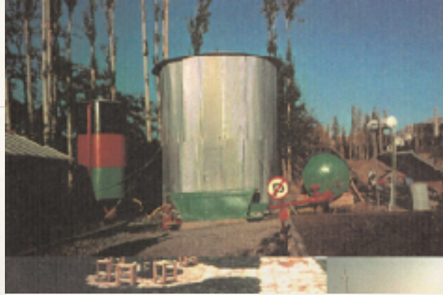
One ton of chicken manure/per day biogas system in Çorum
