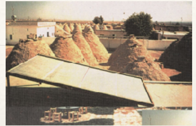
Solar powered interior lighting of Harran Culture House
